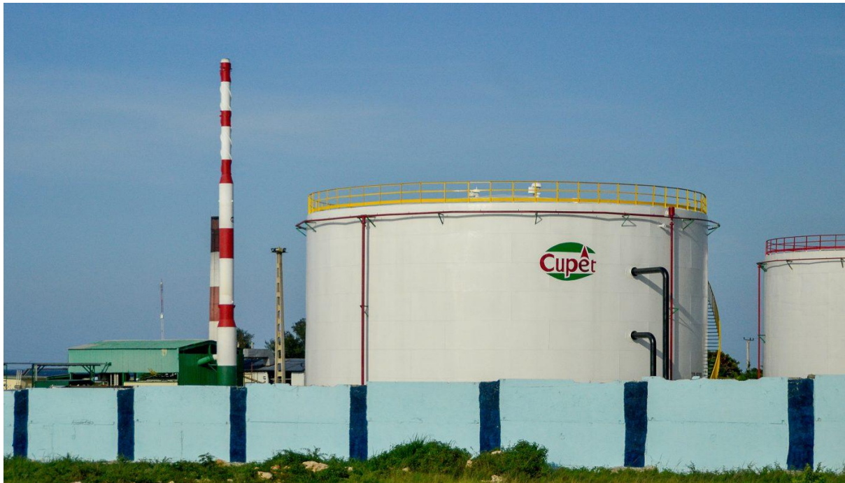
An oil tank belonging to Cupet (source: Mosbatho /Commons/CC-BY-SA 4.0 )
